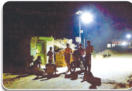
SPV Street Lighting System at a Village
